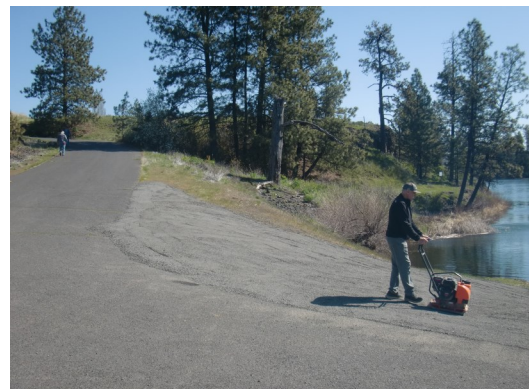
Jeff Pope puts finishing touches on the ramp with the plate compactor.
