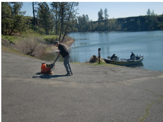
Jeff Pope puts finishing touches on the ramp with the plate compactor.
